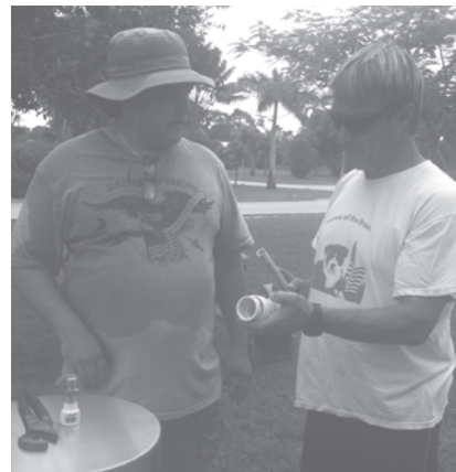
Glen Gareau and Joe Evans installing the new water fountain at the duck pond.
